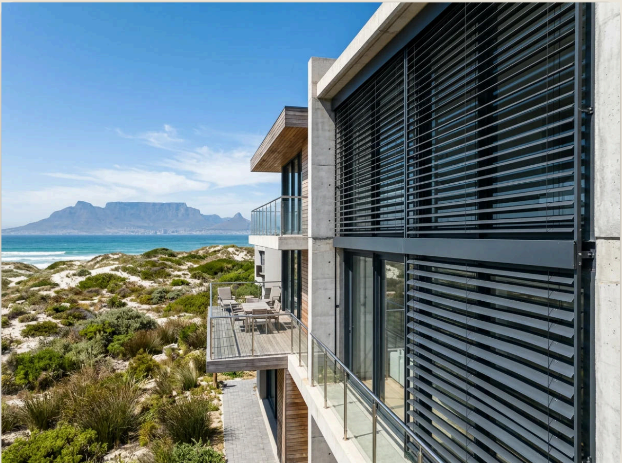
External venetians on a Blouberg facade. The slats are the only part of the shading conversation that can be aimed downward at light coming off the water.
